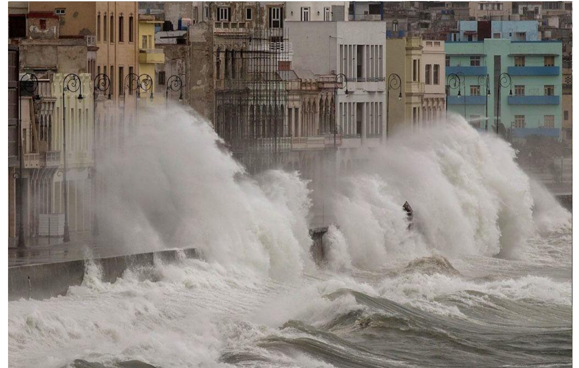
Malecon seawall impact during Irma Image courtesy of Cubadebate / Ismael Francisco
